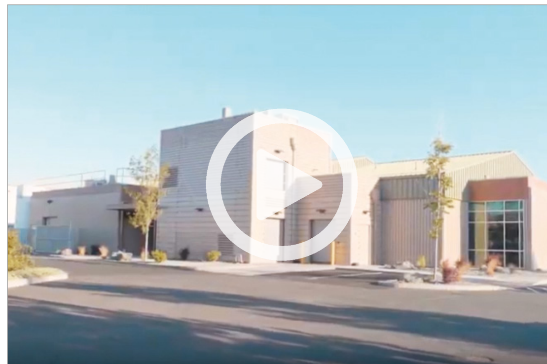
EXAMPLE: Thermo Fisher (Patheon) Bend Facility
